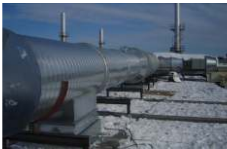
Shoveling snow off the roof made the job at Four Winns more interesting!
